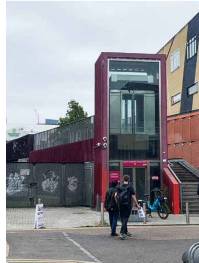
Fig 5.26 Public lift at Hackney Wick, London
